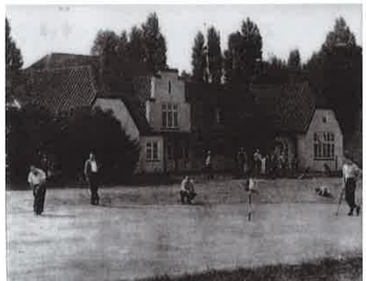
The new clubhouse, later extended.
